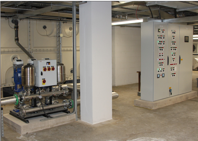
The Dutypoint booster set in the Racecourse plantroom
